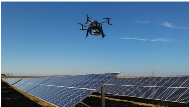
Fig. 1. Photovoltaic plant in Spain with fixed 2V layout structure where aerial thermography is being carried out using a quadcopter equipped with a thermographic camera and a visual camera.
