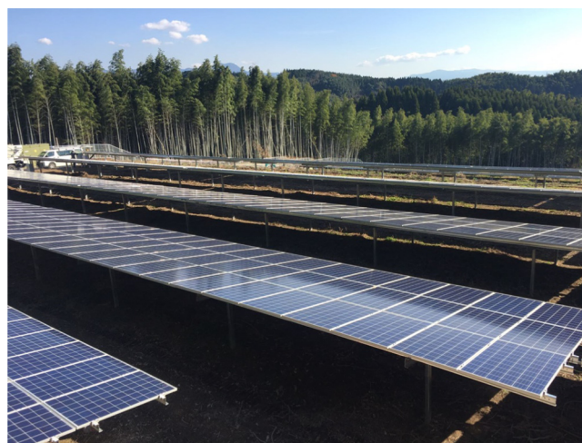
Fig. 7. Photovoltaic plant located in Japan with very low inclination of modules. This module layout complicates the performance of manual thermography as it is difficult to reach the tops of the modules with the necessary angle.
